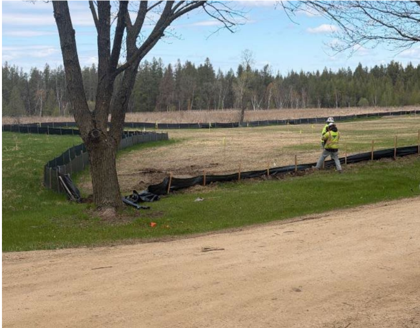
Facing west near MP 2.39, InterCon installing silt fence
