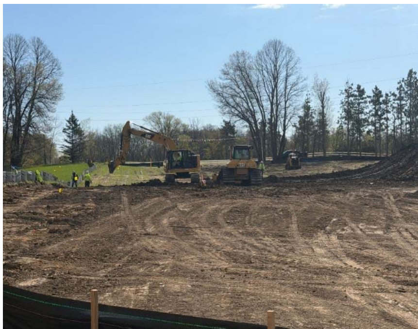
Facing east near MP 2.35, InterCon commencing topsoil removal
