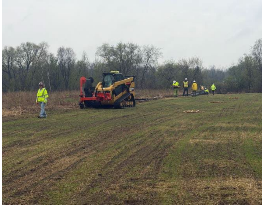
Facing west near MP 3.4, InterCon installing silt fence
