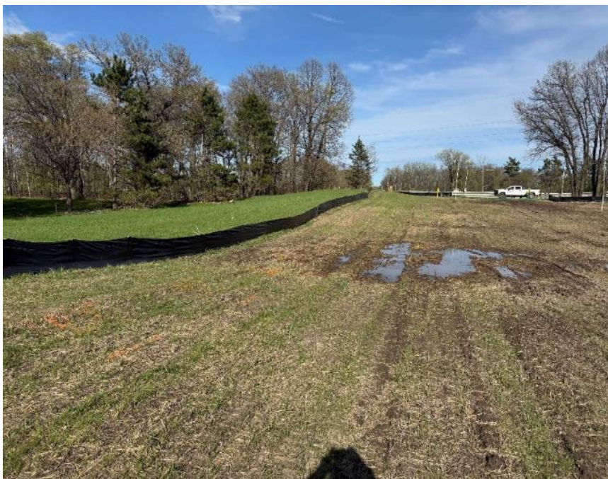
Facing east near MP 2.35, silt fence installed prior to removing topsoil
