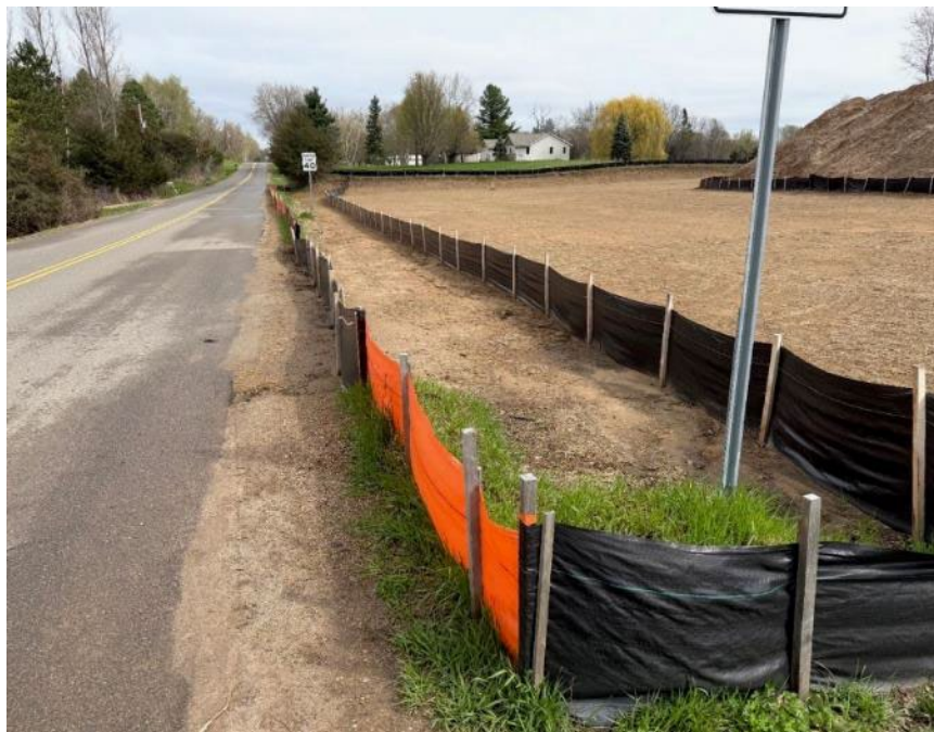
Facing north near MP 1.0, silt fence functioning properly after repairs
